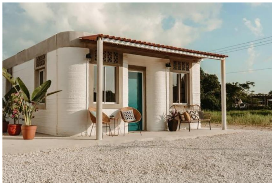
Figure 1. Example of one story 3D-printed construction (Source: [12]).
